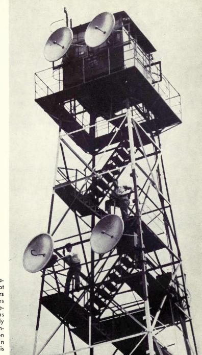
Radio relay stations with 10-foot "dish" reflectors on both sides pick up the television programs and automatically relay them to another relay station or to the main transmitter if it is within range.
