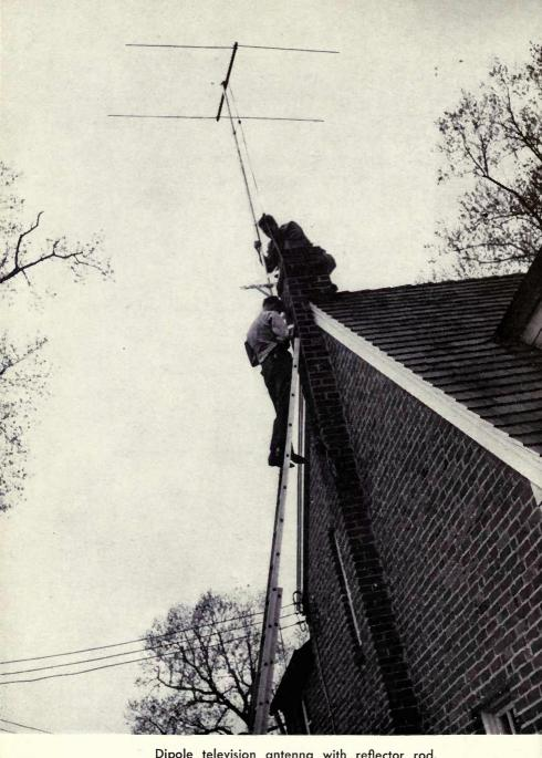
Dipole television antenna with reflector rod.
