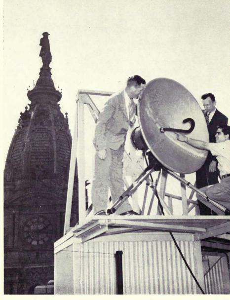
A parabolic reflector, popularly called a "dish," is used to reflect television's microwaves in much the same way that a searchlight projects a beam. The microwave transmitter is contained in a weather-proof cylinder attached to the back of the parabola.
